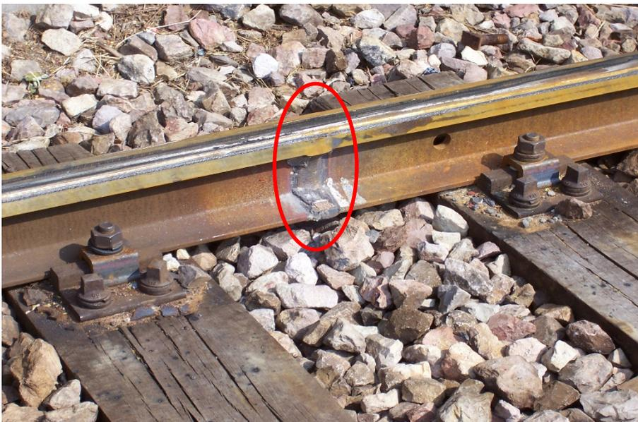
Figure 4.7 Welded rail joint[69]
