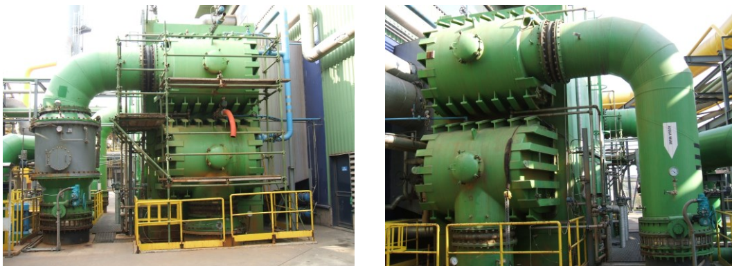
Figure 3-3: Pictures of the heat exchanger at Servola power plant: inlet (left side) and outlet (right side).
