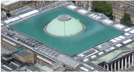
Canopy of the great court of the British Museum. The steel gridshell follows a triangular mesh.
