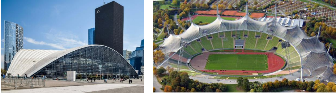
Figure 1 Double curvature structural envelopes. Left: The concrete shell of the CNIT, Paris (©Alexandre Prevot). Right: Cable net of the Olympic Stadium, Munich
