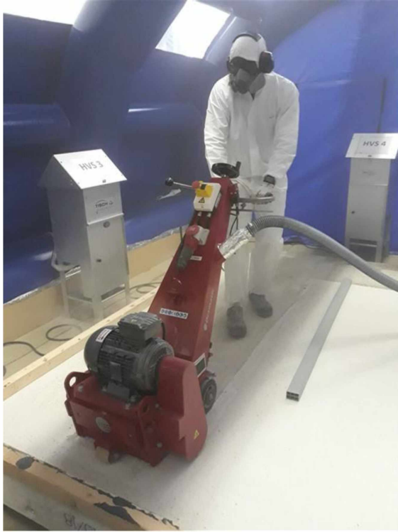
Figure 4 - Dust perceptible to the naked eyes along with a milling ride; on the back right, the connecting pipe to the vacuum is distinguishable
