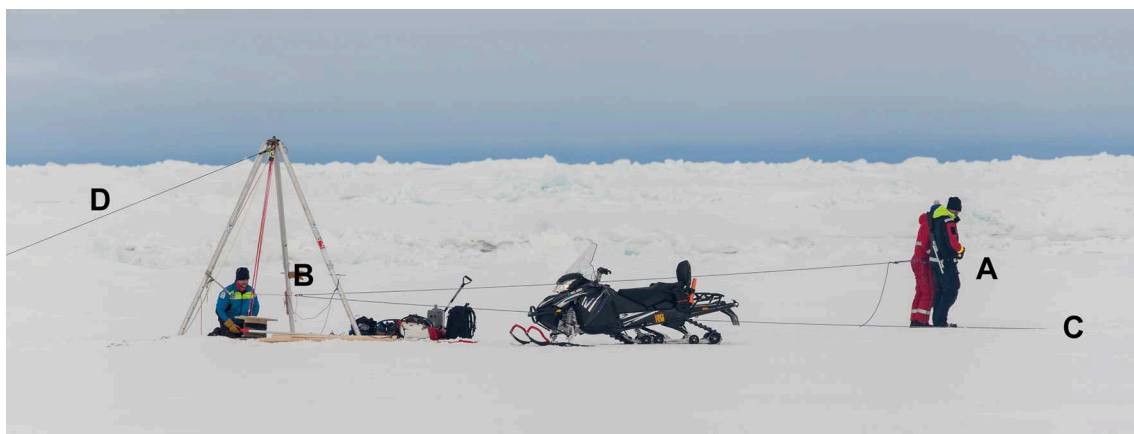
FIGURE 6 | Overview of the recovery procedure. Two persons (A) pull up the load with the 2:1 pulley system. The loop pulley rope is fixed in the ground (C) and diverted in the multiplier block (B). Note the guy rope (D) that is necessary to keep the tripod from tipping over. Picture was taken during the training session, where a bigger tripod was used. No Skidoo was available during the actual recovery.
