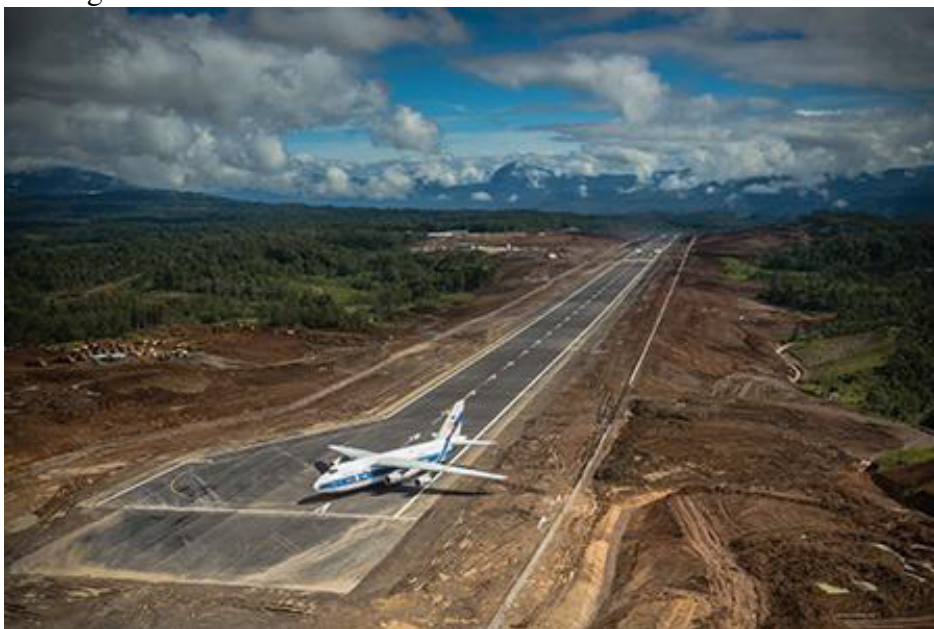
Figure 4 - Komo Airfield (Source WT Partnership website, http://wtpartnership.com.au/our-team-experience/png-lng-komo-airfield-png/ ).
