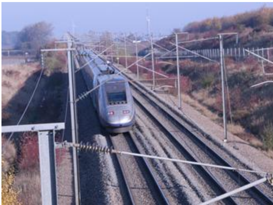
10 11 12 13 14 15 16 17 18 19 20 21 22 23 24 25 26 27 28 29 30 31 32 33 34 Fig. 1. Catenary line, pantograph and rail return current to feed the train electrical traction chain.
