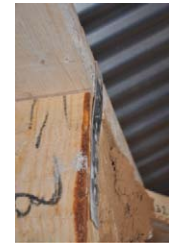
(i) GUA 390%: Connection– Location 4: West shear wall
