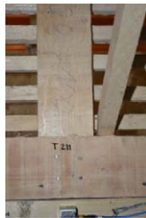
(c) HTI 200%: Roof bracing– Location 1: South transv.wall
