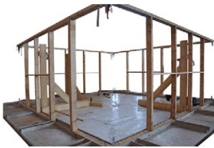
(a) Timber structure anchored into the steel frame
