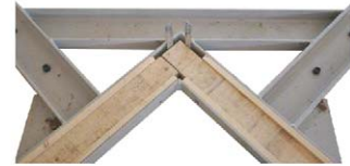
(c) Mudsill locked by a wooden wedge
