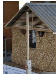
(h) GUA 390%: Filling Location: South transv.wall
