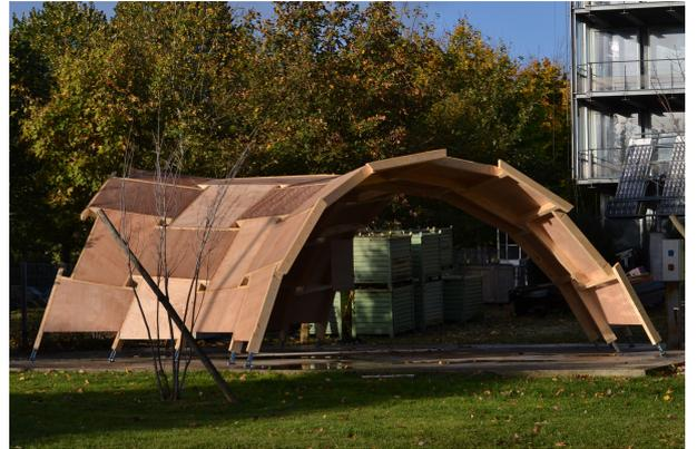
Figure 19: Timber pavilion using the principle of hybrid nexorades (copyright: Romain Mesnil).
