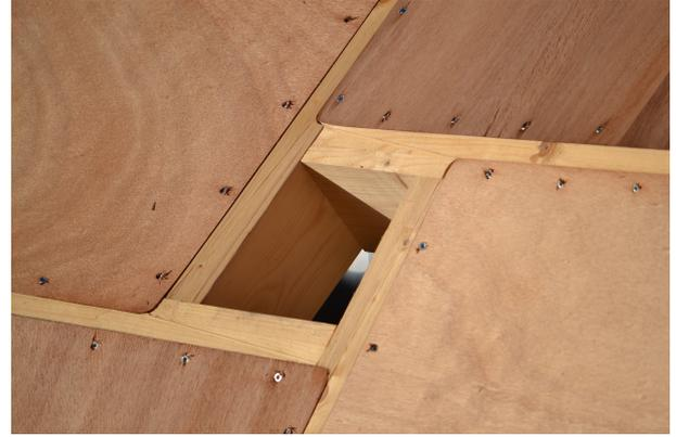
Figure 22: Attachment between flat panels and members, (copyright: Romain Mesnil).
