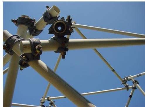
Figure 1: Simple two-valent connections in a nexorade (picture: [6])
