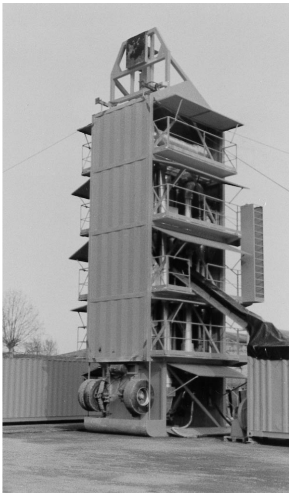
Fig. 4. Photograph of the main truck.
