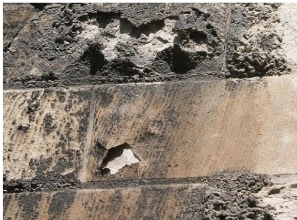
Fig. 2. Formation and eruptions of blisters on the Lede stone surface (Saint Bavo's Cathedral, Ghent, Belgium).
