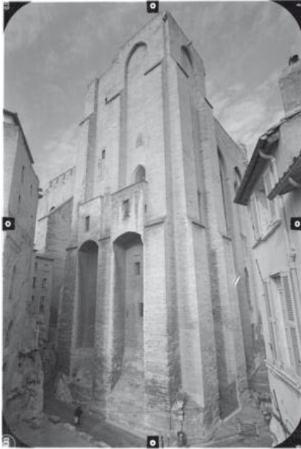
Tour Saint-Laurent south-east overview
