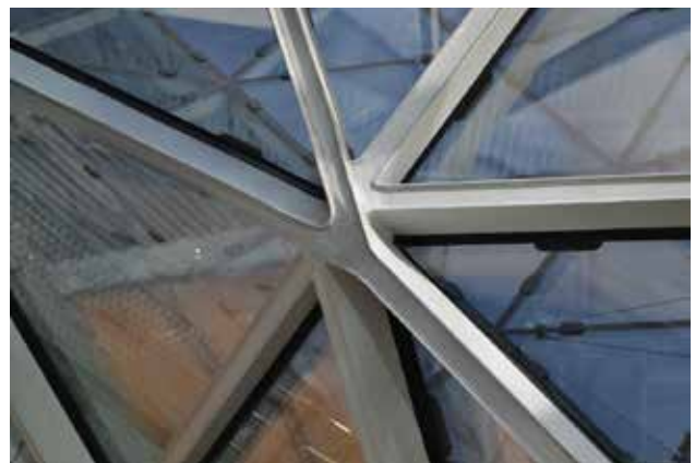
Figure 1: A node with torsion (picture: Romain Mesnil)
