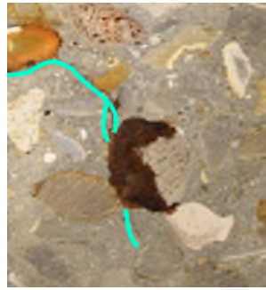
Fig. 14 Experimental crack pattern
