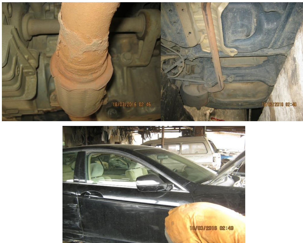
Fig. 29. Corrosion Effect on Different Parts of the Underneath of a Car (Manufacturer: HONDA Model: ACCORD 2.0 LX, Year of Manufacture: 2008).
