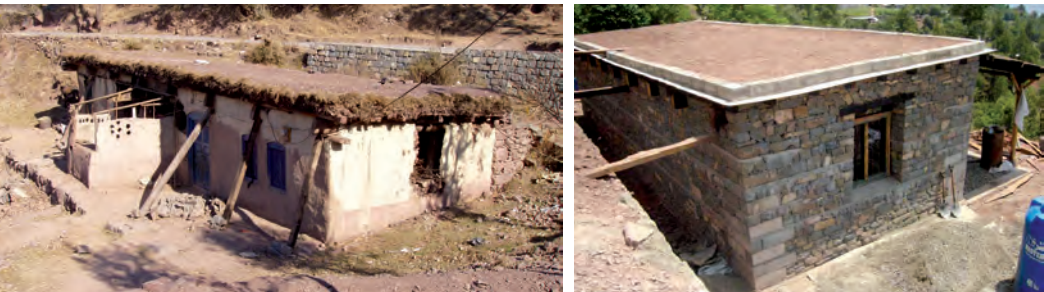
Pakistan, after the 2005 earthquake: damaged house and newly rebuilt house with improved stone masonry
