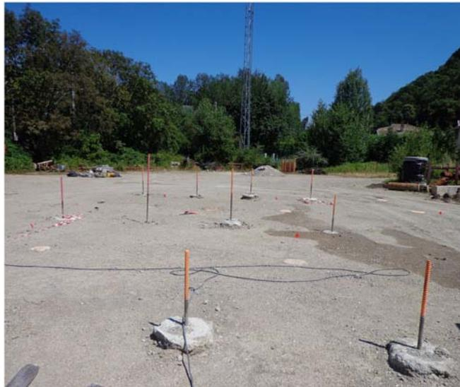
FIG. 8. Photo of a soil reinforced with columns of concrete 0.4m in diameter and 15m in depth (Courtesy of M enard).
