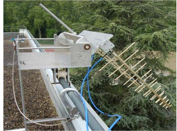
Fig. 2. Mounting of the antennas on the roof.
