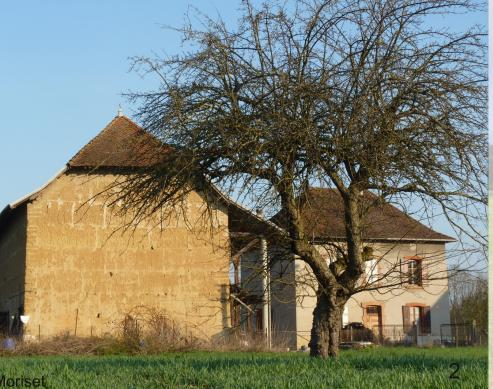
**Rammed earth building** involves compacting layers of earth into a formwork to create walls (pict.2). Widely used in Rhone-Alpes region before it declined after the Second World War, the technique has turn in the last decades to be promoted by a wide range of actors, from architects and researchers to craftsmen, inhabitants, politics or even materials producers.
