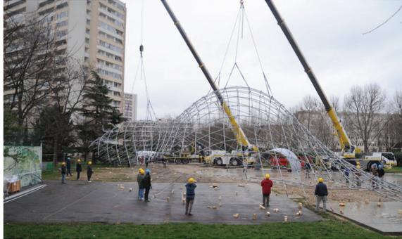
Figure 2: Grid erection with large deflections
