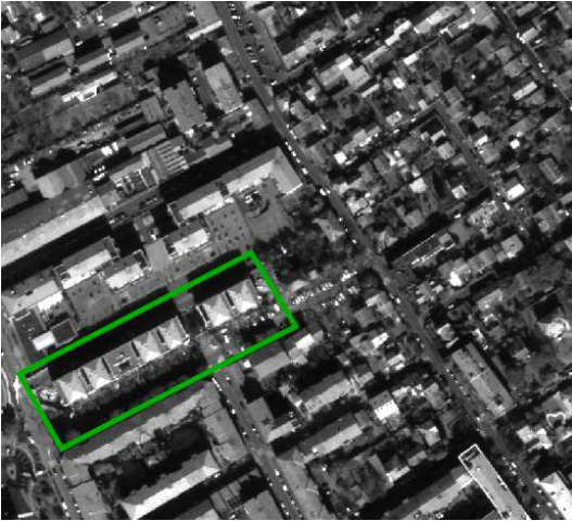
Fig. 1. Example of a pair of optical satellite images, with an apparent change surrounded in green (construction of a building). Both images have a resolution of 50cm and an incidence angle close to nadir, but they have been acquired by different sensors (Geoeye and Worldview).
