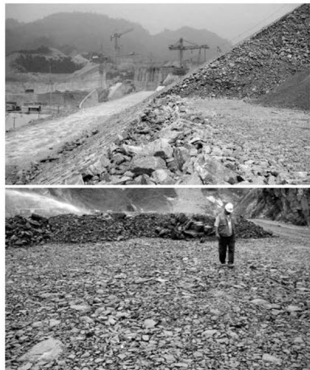
Fig. 1. Typical rockfills used in dam construction
