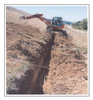
**Figure 5.** Digging up of the trench for optical fiber installation along the dike.
