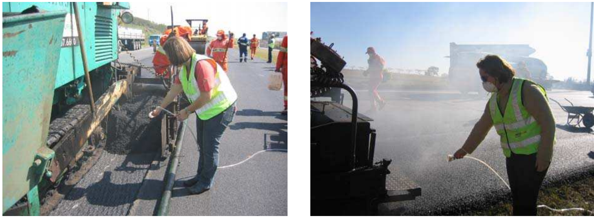
Figure 2: Reduction in visible emissions when paving WMA (left) and HMA (right)
