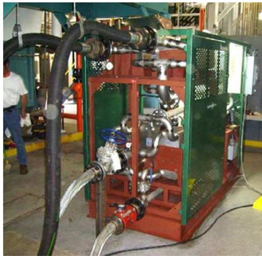
**Fig. 8.** ElectraTherm green machine with patented twin screw expander
