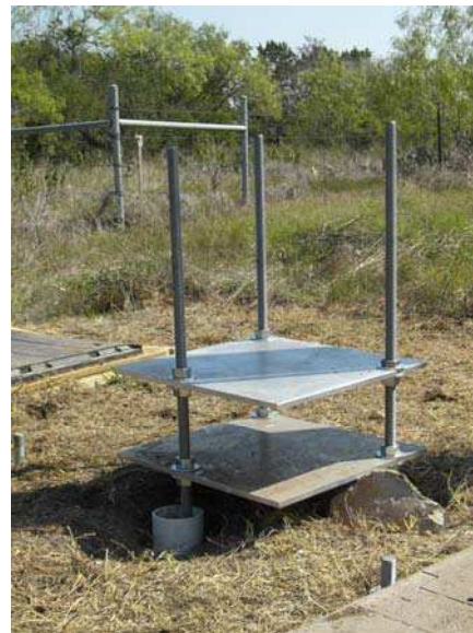
Figure 5. Edwards Aquifer field site monument installation. Plates and long rods were removed after the epoxy cement had cured. Shorter rods were installed and the plates were replaced to form bracing for the vertical rods. Finally, aluminum pillars were threaded to the top of the steel rods, and E2 lowered onto them. The last step involved erecting the instrument shed around E2.
