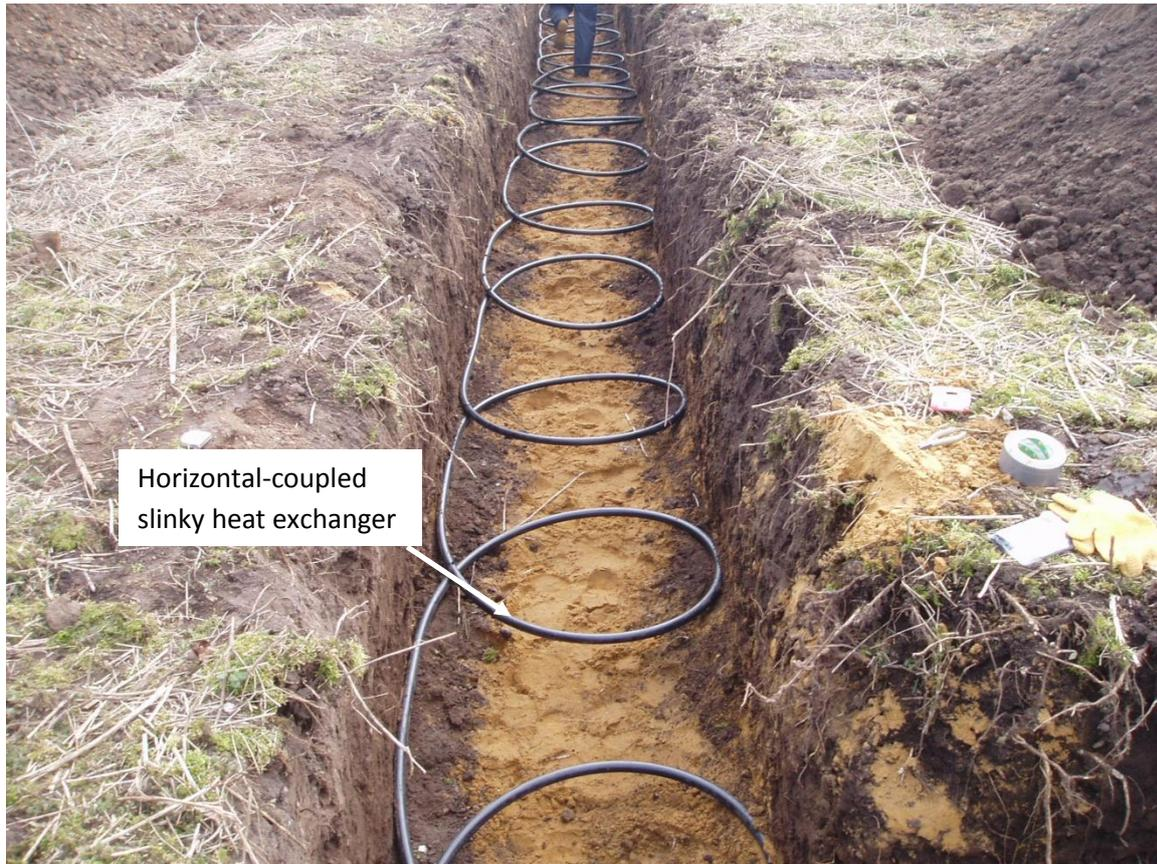
Figure 1 Image of the horizontal-coupled ground source heat exchanger at Talbot Cottage, Drayton St Leonard site, Oxfordshire, UK
