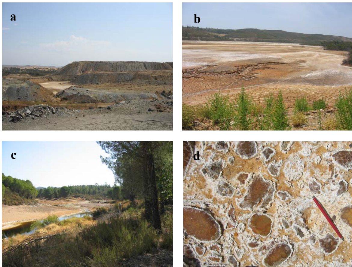
Figure 11. (a) Panoramic view of terraced mine dumps on the Las Herrerias mining site. (b). Drainage with oxidized crusts developed on a surface of hydrated sulfate on the mill tailings dam of the Sotiel-Almagrera mine site. (c) View of sandbar development on the Odiel River, with coarse boulders on the sands, rimmed by white crusts of hydrated sulfate at the edge of the water. (d) Development of white hydrated iron sulfate crusts over oxidized boulders from sediments taken from the Odiel River.
