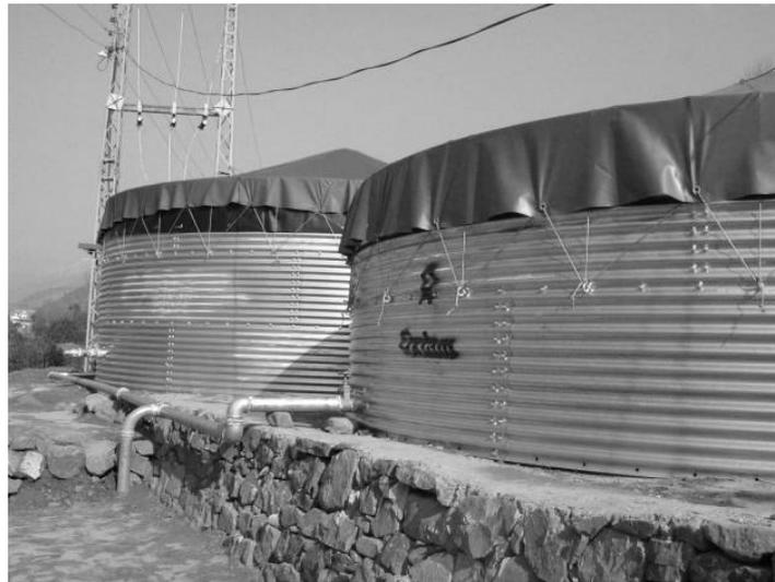
Figure 3: Emergency batch sedimentation tanks used in Gahri Dupatta.
