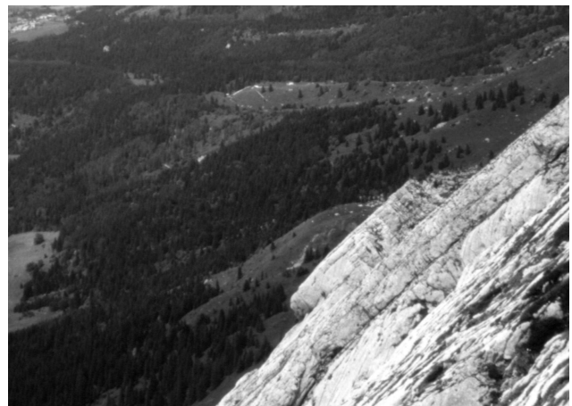
Figure 1. A potentially unstable rock mass of about 10,000 m 3 . The slab is 6 m thick. The potential failure mechanism is a plane slide.
