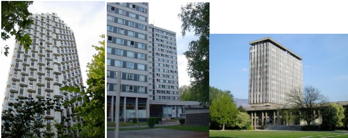
Figure 2: The Mont-Blanc Tower, the ARPEJ Tower and the City Hall
