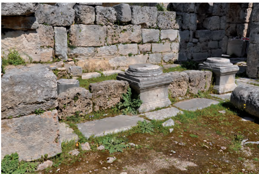
Fig. 36. Church at Karian Kaunos with stone barriers separating the nave from the aisles.
