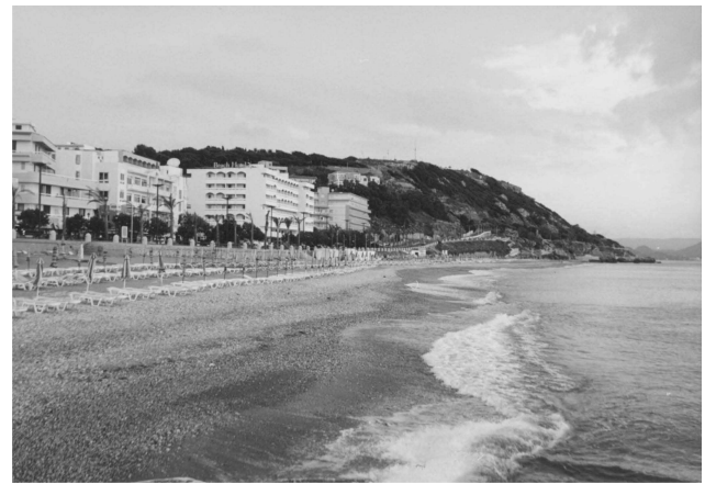
Fig. 3. View of the coastal segment of the city of Rhodes inundated by the local tsunami of 24 March 2002.
