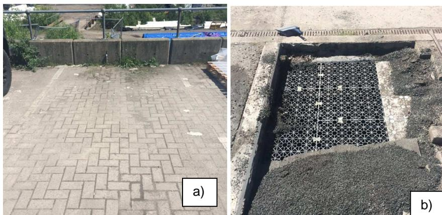
Figure 2. a) Interlocking porous paving car park bay excavated for this study from Bury. b) Excavation of the car park bay exposing the profile of a porous paving system.
