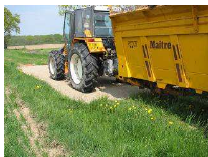
Photo 9 Passage of spreader in the gravel pit
