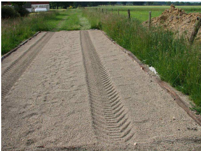
Photo 6: Gravel pit after passage of spreader
