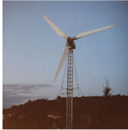
Figure I.5 : Eolienne de 10 kW [I.10]
