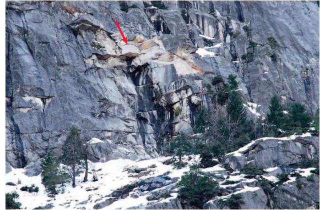
Fig. 4. Photograph of Staircase Falls rock-fall detachment area taken 21 days after 26 December 2003 event, showing light colored joint-controlled detachment surfaces. Rock debris impacted snow-covered ledge immediately below source area, and then fell \sim 745\text{ m} down joint-controlled ledges to Yosemite Valley floor. Note heavy dark drainage paths below detachment area indicating water flow through joints. Overhanging rectangular block in center left of photograph (marked by red arrow) fell during 9 June 2007 rock fall. (Photo by Dan Horner, NPS).
