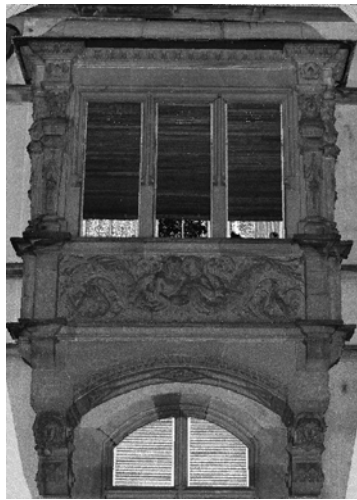
Fig. 15. Detail of the façade (grey scale intensity image), 1 point / 1cm
