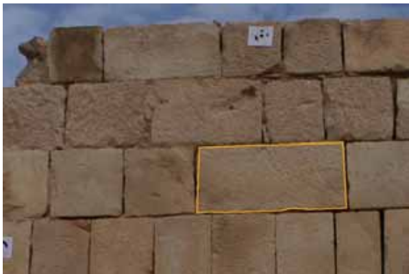
Figure4: A block perimeter easured with Arpenteur
