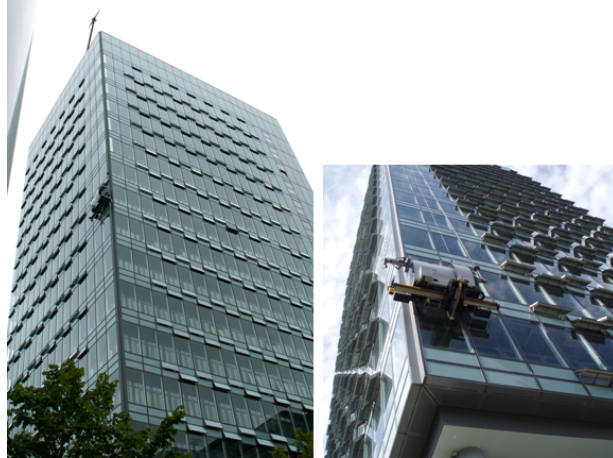
Figure 7: SIRIUSc on the high-rise building of the Fraunhofer-Gesellschaft's headquarters in Munich
