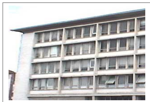
Figure 1. Photograph of the building under study
