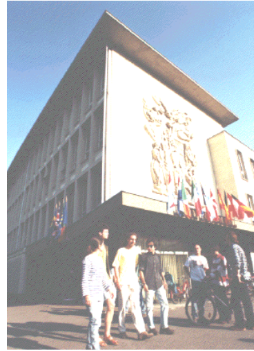
Figure. 4. Test building (ENSAIS)
