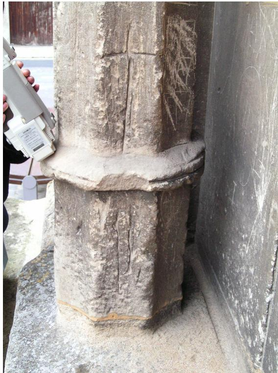
**Figure I-27.** Engravings in the soft Lutetian limestone used in the Neuville-sur-Oise church, Val d'Oise, France.
