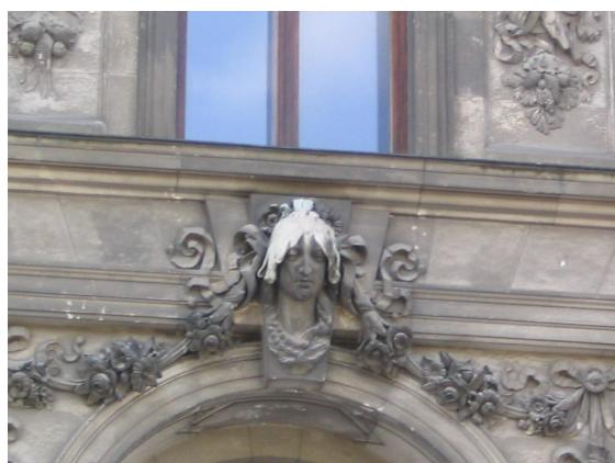
**Figure I-9.** Erosion by water streaming of the carved part of the soft stones exposed to rain, Hofburg, Vienna, Austria (limestone).
