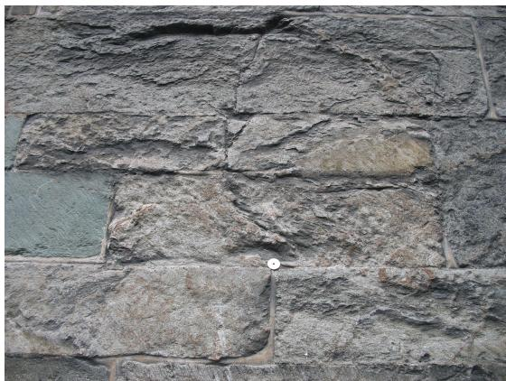
**Figure I-7.** Granular disintegration due to freeze and thaw on the Nidaros Domkirke, Trondheim, Norway (schists).
