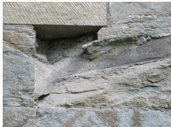
**Figure I-8.** Contour scaling due to freeze and thaw on the Nidaros Domkirke, Trondheim, Norway (schists).
