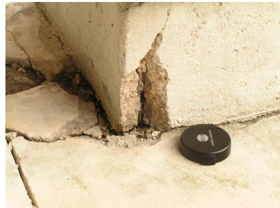
**Figure I-15.** Salt weathering in concrete, Neuville-sur-Oise, Val d'Oise, France (concrete).
