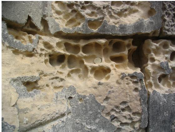
**Figure I-5.** Honeycomb weathering on St Etienne church, Fecamp, Seine-Maritime, France (limestone). This church is located 300m of the sea
