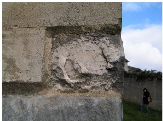
**Figure I-21.** Alteration due to inappropriate restauration on Villiers-Adam church, Val d'Oise, France (limestones).
