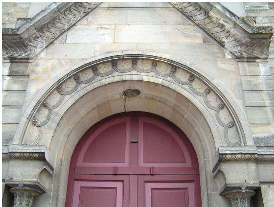
**Figure I-25.** Cracking due to mechanical load on the arch above the main door of Neuville-sur-Oise church, Val d'Oise, France.
