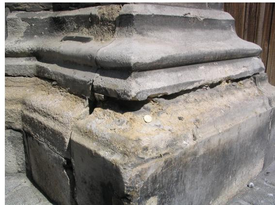
**Figure I-4.** Granular disintegration on Stefansdom, Vienna, Austria (sandstone).
