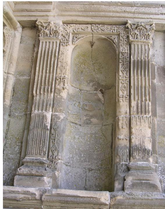
**Figure I-26.** Cracking due to mechanical load on an alcove. Guiry-en-Vexin church, Val d'Oise, France.
