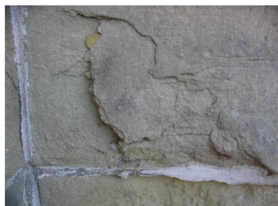
**Figure I-2.** Contour scaling on church of Objat, Corrèze, France (sandstone).
