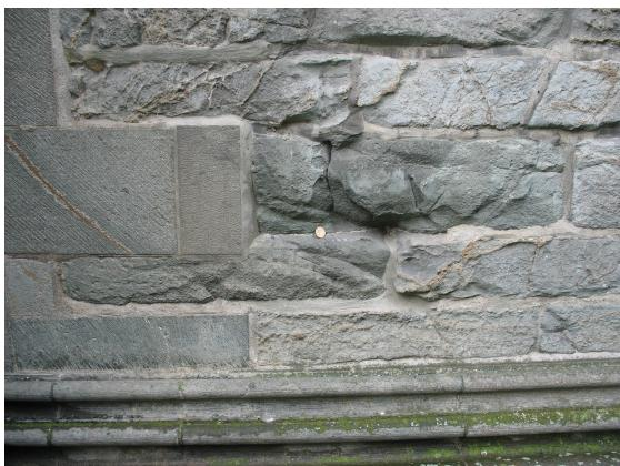
**Figure I-20.** Alteration due to inappropriate restauration on the Nidaros Domkirke, Trondheim, Norway (schists).
