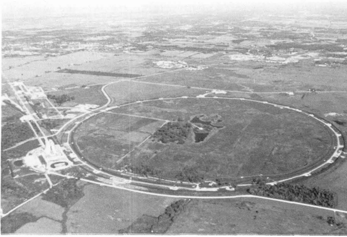
Fig. 6 : View from the air of the Fermilab site showing the 1 kilometer radius circle below which the accelerator is housed ( \sim 1977 )
