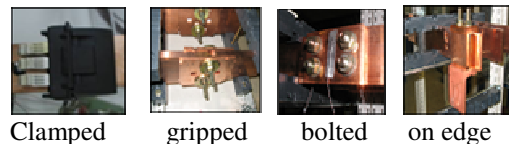
Fig 3 Different types of electrical joints.
